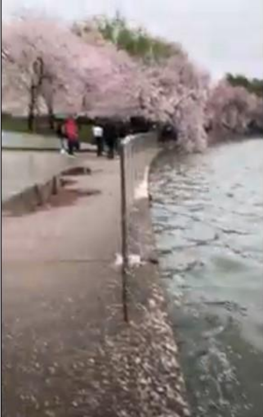
The seawall shoreline at the MLK Memorial. There is standing water and water nearing the top of the seawall. 3.25.23
